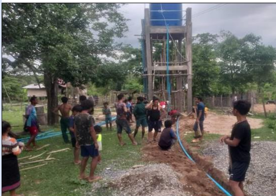
VDCs members and villagers together construction water system in Xuong Yai village (April 2019) © MCNV
